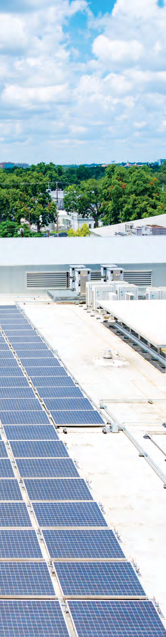
Rooftop Solar Installation
